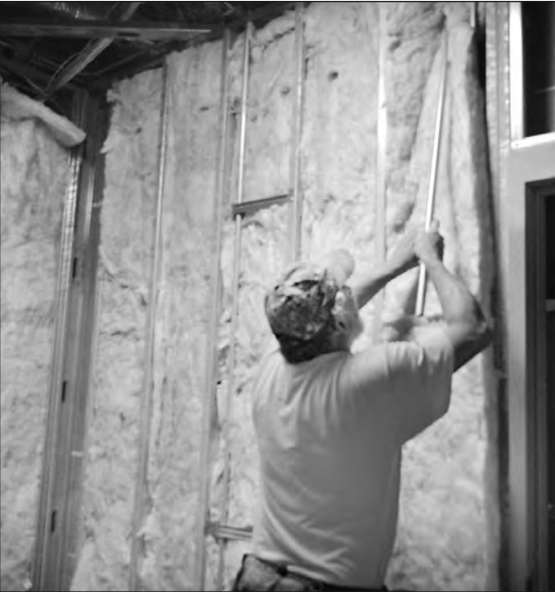
THE CRITTENDEN PRESS Ronald Calhoun of Princeton Lumber Co. works Monday afternoon installing insulation inside a revamped office at Crittenden County High School.
